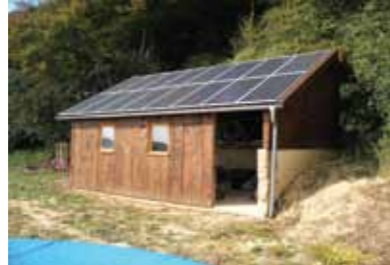
▲ 1MW project in Macedonia
