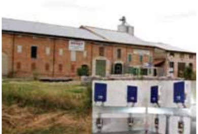
◀ 102kW project in Italy
