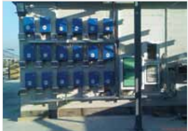
10kW rooftop project in Daufenbach, Germany
