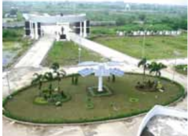
▲ 125kW project for school in Surabaya, Indonesia
